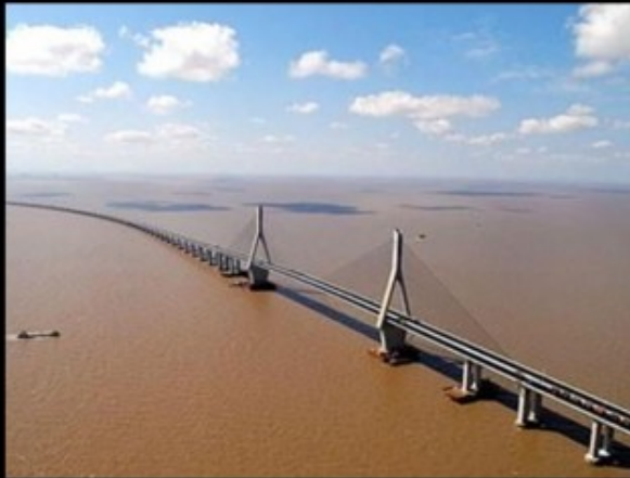
Hangzhou Bay Bridge
