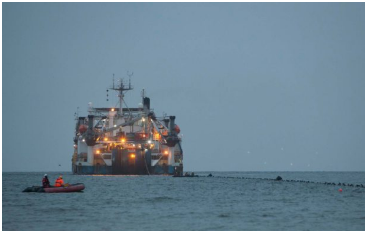
Western Link marine cable landing at Ardnail Bay. Picture by Chris James
