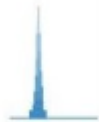
The highest building in the world, Tower of Dubai, is 818 m high
