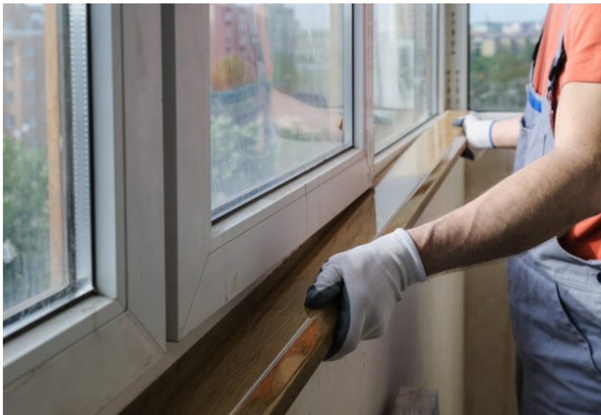
Worker is installing a window sill on a polyurethane foam.
